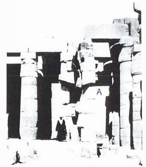
Fig. 127. Remains of a hollow wall in the Ramesseum, showing the poor quality of the masonry. A surplus half-drum of a column has been used at A
