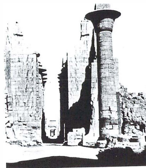
Fig. 69. Column of King Taharqa at Karnak, leaning from the vertical owing to the settling of its foundations. It has recently been taken down block by block and rebuilt
