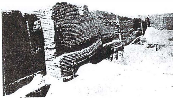
Fig. 254. Brick girdle-wall at Abydös (Kôm el-Sultân), showing sections laid alternately on concave and level beds
