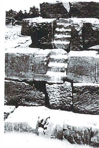
Fig. 211. Remains of a stairway in the pylon of Tuthmosis III (Pylon VII) at Karnak
