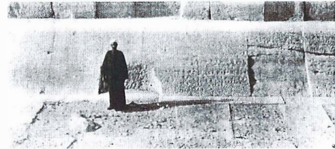
Fig. 96. Casing-blocks on the north side of the Great Pyramid. The joints in these blocks do not gap more than \frac{1}{16} " at any point in their surfaces. Behind are the 'packing-blocks' of the second course
