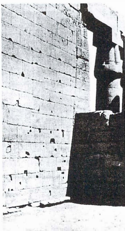
Fig. 102. Masonry with blocks of unequal heights. Temple of Amenophis III at Luxor, east side
