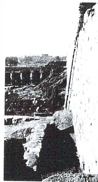
Fig. 234. The unfinished pylon (No. 1) at Karnak, from the north-east, showing remains of the constructional embankments
