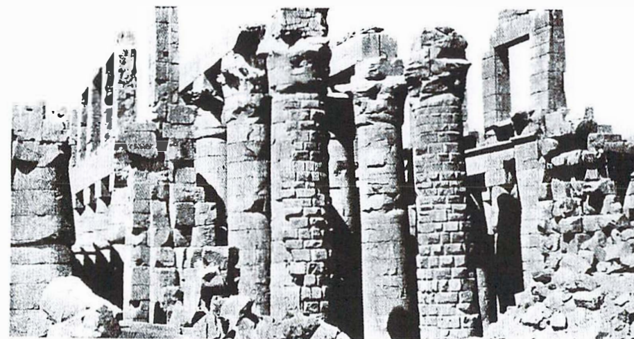
Fig. 166. East end of the Great Hall at Karnak, showing ancient repairs to the columns
