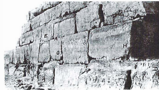
Fig. 97. South face of a mastaba at Giza. The levelling of the casing-blocks, which have now disappeared, was carried, at AB and CD, a short way into the core-blocks. At EF and GH, traces of the levelling of the intermediate casing-blocks can be seen. The core-blocks are about four feet high
